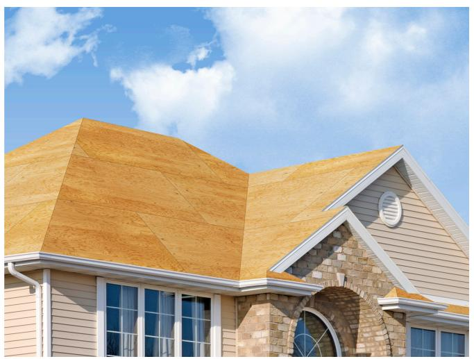
A good roof deck is the foundation for the rest of the roof. If your existing deck is damaged in any way, your contractor will need to replace those boards in order to insure the integrity of the remaining system components.
